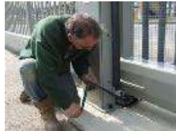
'**Fail Release**' is when the system or operator is set up to allow reversal during a power failure or system fault. This means the gate may be used manually without the need to release the mechanism/operator from the gate.
